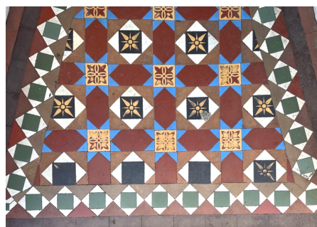
There are a few true encaustic tiles in this Morningside Road shop doorway, worn so you can see the working.
