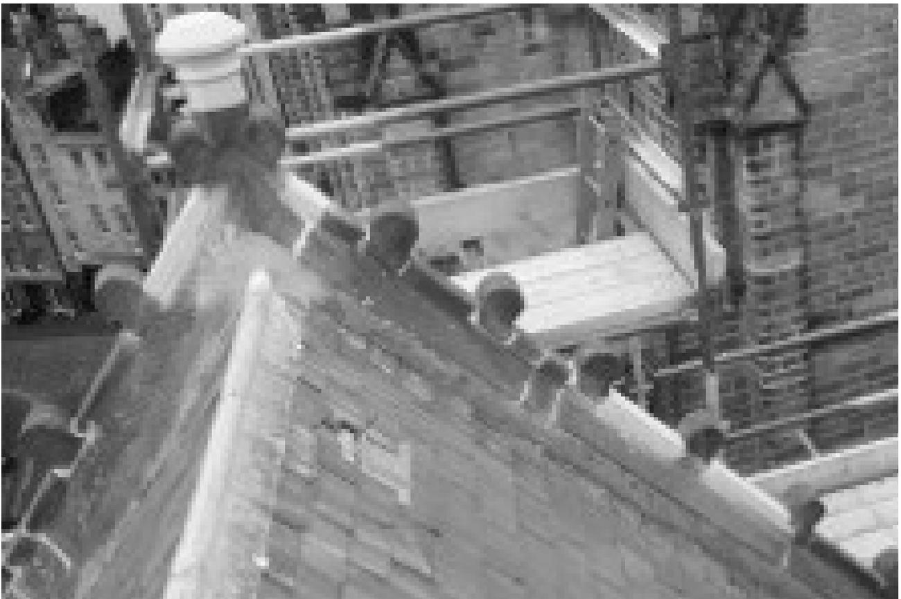
The west gable from above, after work had been completed: the lighter-coloured areas (including the top of the apex stone and the spaces between the third and fifth crockets on the right) are new stonework.
